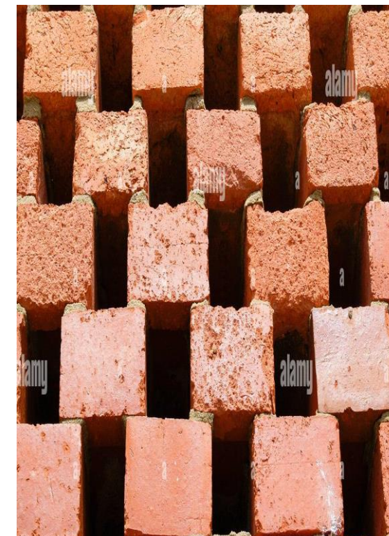
Perforated brick wall with mortar joints (17m to 40m)
